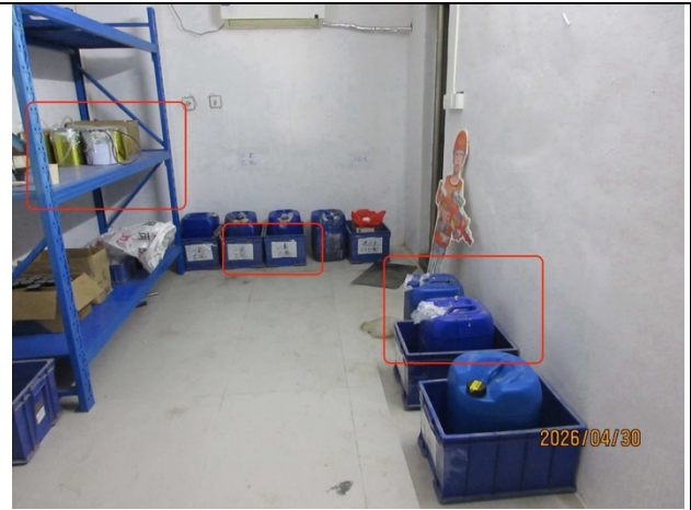
PA 7.7 No secondary containment for chemical in chemical storage area and chemical only with Chinese name label
